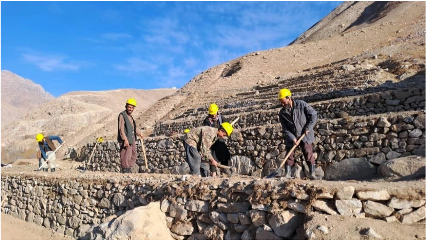
Laborers employed by SFL preparing hillside terraces for tree planting. More than a thousand such terraces have been built. Both the trees and terraces help to stabilize hillsides, preventing erosion and thereby protecting property and lives.
