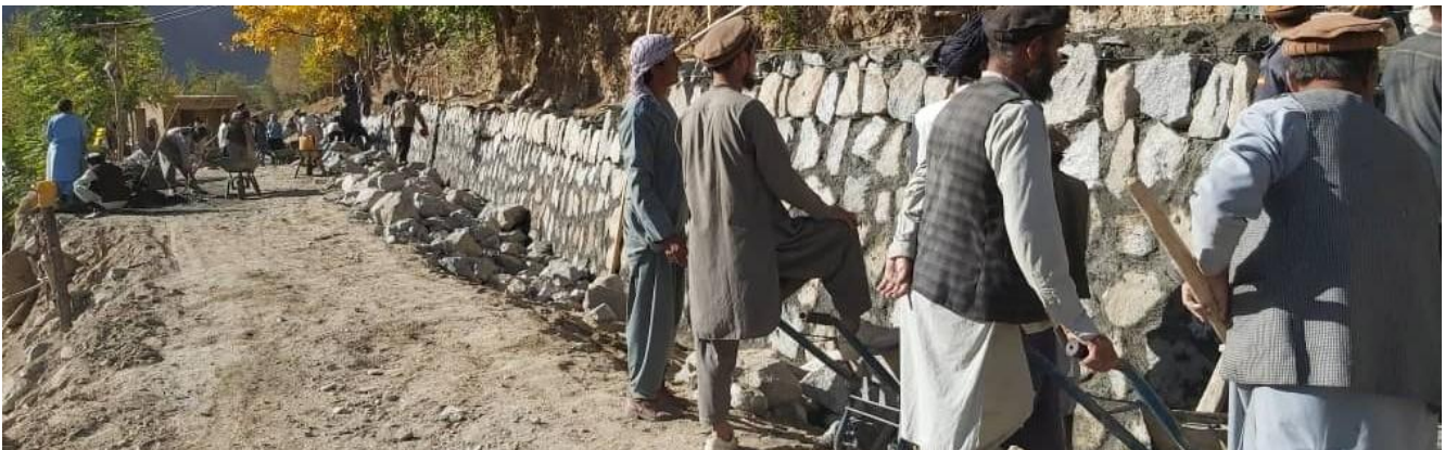
Workmen employed by SFL in Afghanistan building a retaining wall next to a rural road
